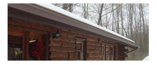
Pictured: Gutter Helmet in the winter with icicles. This home also had heat loss issues enhancing the amount of ice buildup.
